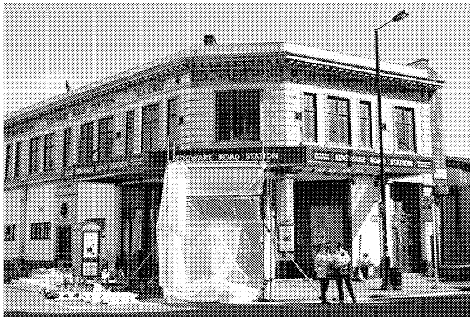
Above: Edgware Road sealed off
